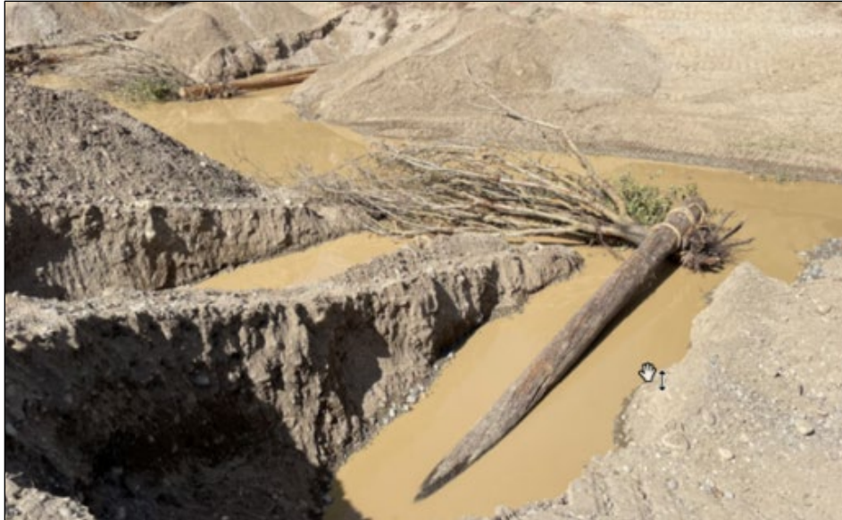
Figure 11: Habitat IWM Anchoring Example
